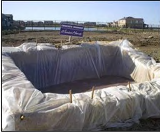
Plate 3-1 Typical concrete wash out areas
